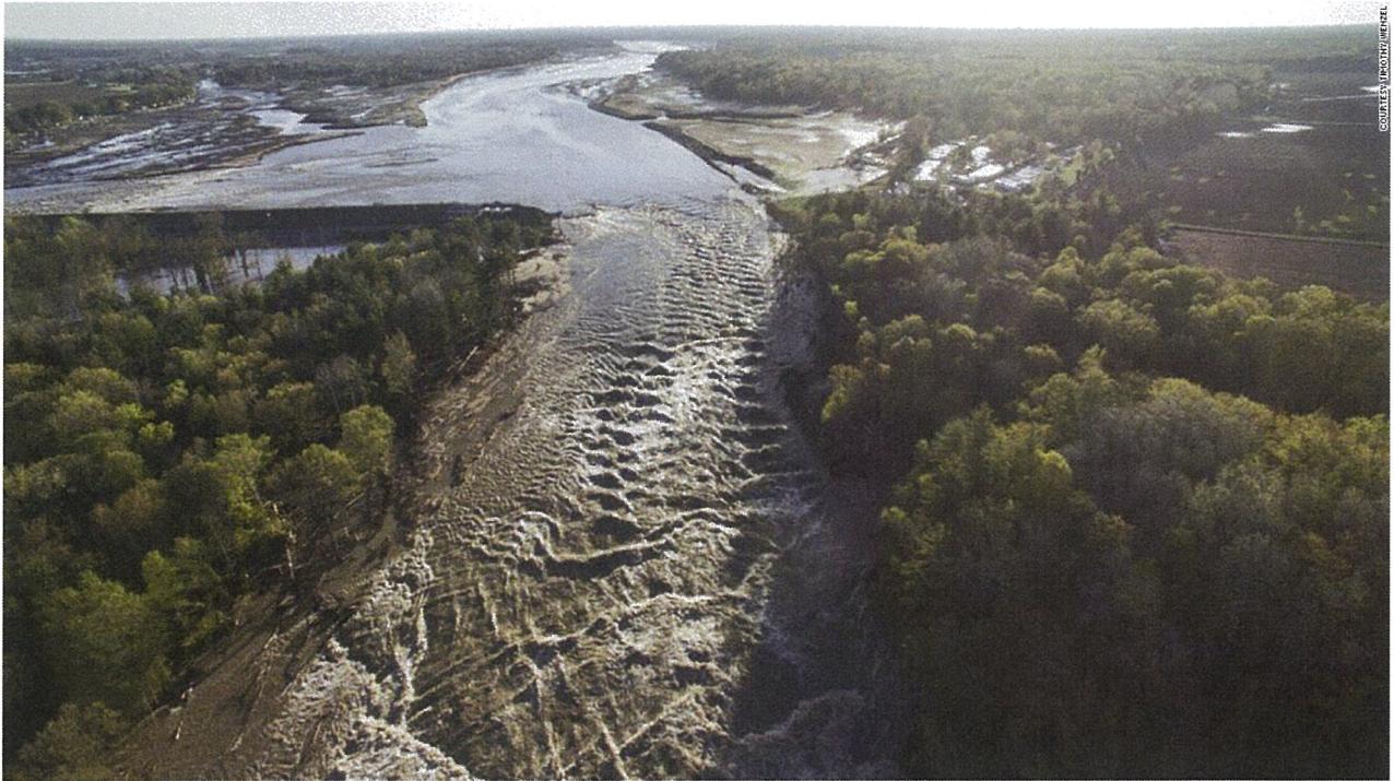
Aerial photo of breaching Sanford Dam, Sanford, MI, Wednesday, May 20, 2020. 63
