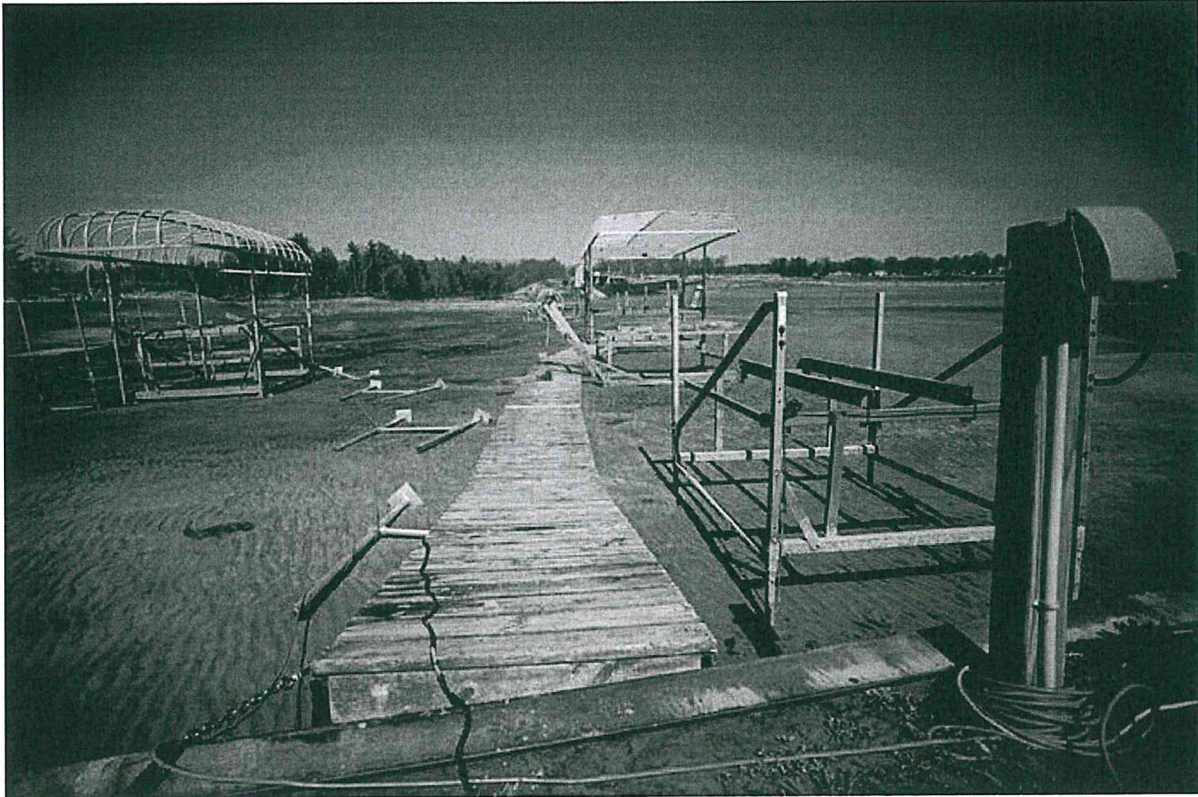
Washed out boating docks on Wixom Lake due to the failure of the Edenville Dam on Wednesday, May 20, 2020. 63
