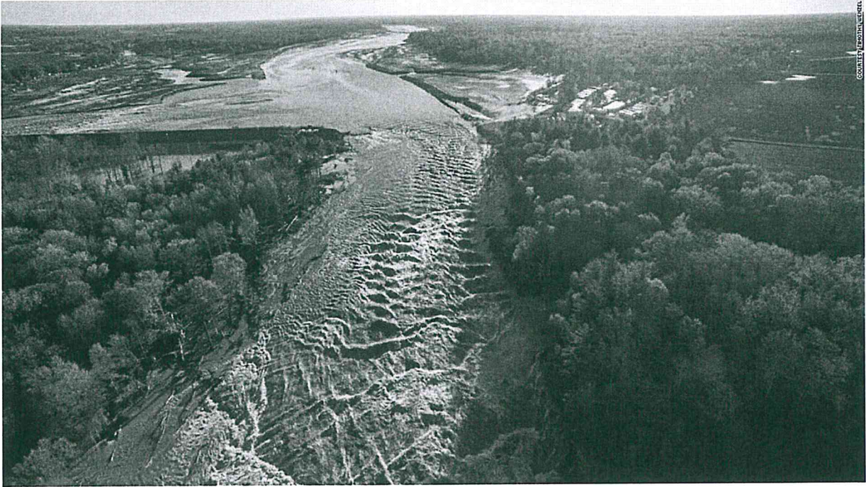
An aerial image taken by a drone shows the Edenville Dam breach on Wednesday, May 20, 2020. 59
