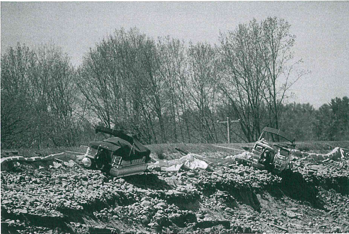
Two boats sit atop what remains of the Edenville Dam, washed up after severe flooding on Wednesday, May 20, 2020. 64
